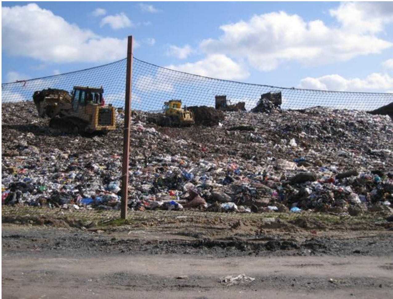
Heathfield landfill site shows bulldozers moving trash and garbage into a landfill with netting (required by EPA guidelines) to prevent waste from blowing away. (Stott, 2010)
